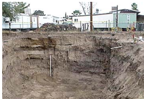
Excavated Soil from the Former E. C. Winter Property
