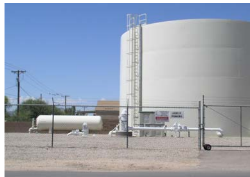
Flowing Wells Irrigation District Water Tank
