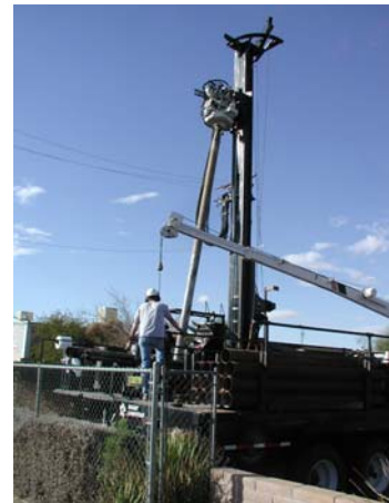
Installation of Monitor Well at Site
