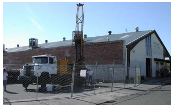
Groundwater Monitor Well Being Installed near Historic Dry Cleaners
