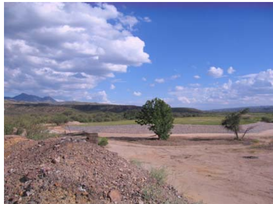
Completed Erosion Protection and Clean Cap on Upstream Tailings Pile
